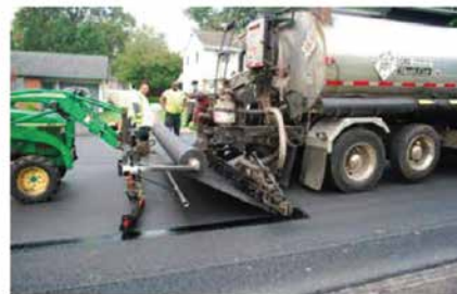
The paving fabric distributor truck sprays PG 64-22 sealant followed by placement of the paving fabric by the spreader/broom tractor unit.
