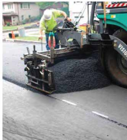
9.5-mm hot-mix asphalt is placed over the paving fabric.
