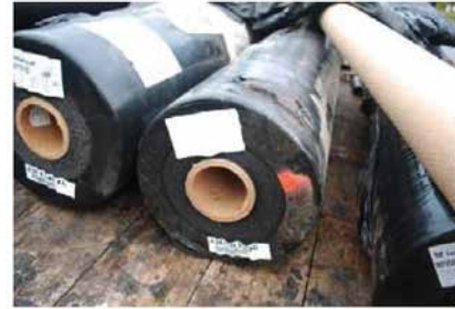
Geotextile rolls must be stored off the ground and adequately covered to protect them.
