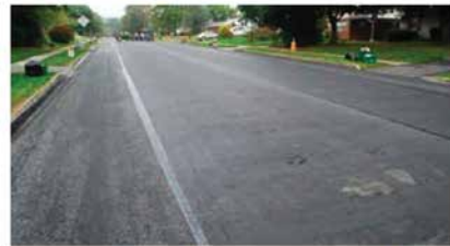
The paving fabric is placed over a leveling course, which is done the previous day to allow the roadway to cool prior to applying the sealant and paving fabric.
