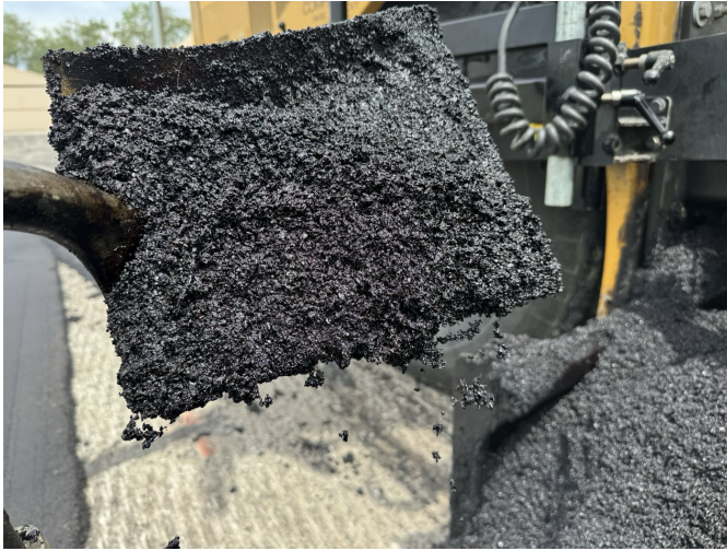
ACE XP fiber-reinforced mix at the paver (double dose).
