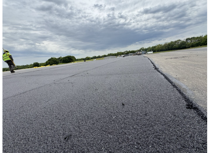
New overlay lift placed over the ARMI interlayer — paving in progress.
