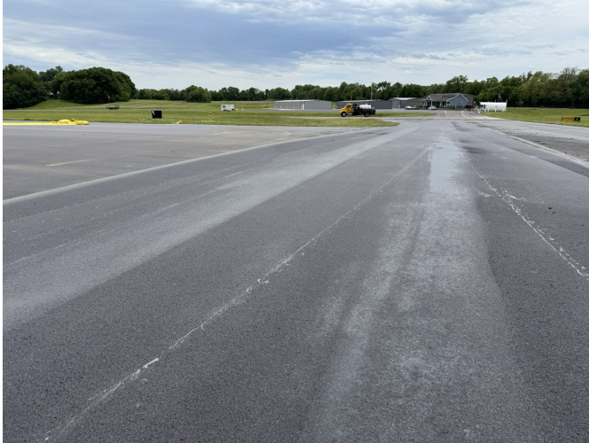
Completed ACE XP runway surface looking toward the apron and hangars.
