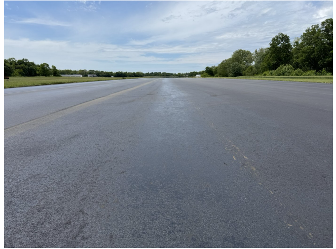
Smooth, crack-resistant runway after final placement.
