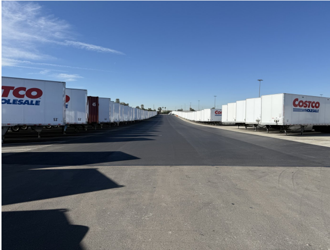
The completed trailer yard in service — loaded trailers staged on the new reinforced pavement.
