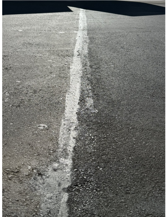
Pavement transition at the edge of the new reinforced section.
