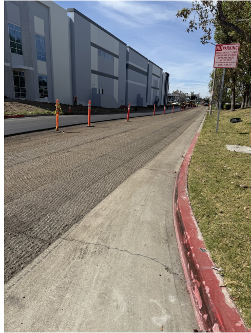
The graded corridor before paving — curb to curb preparation complete.
