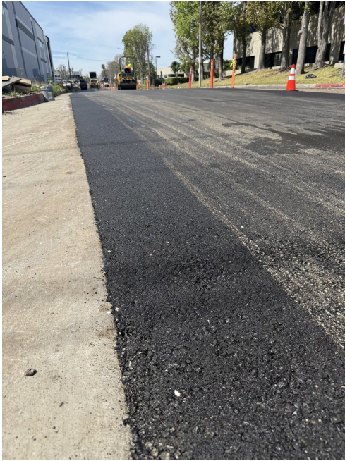
New ACE XP-reinforced pavement fronting the industrial development.
