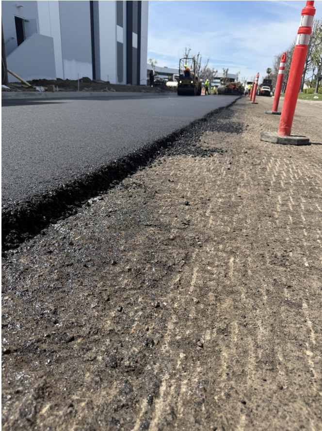
The new reinforced lane taking shape alongside the prepped subgrade.
