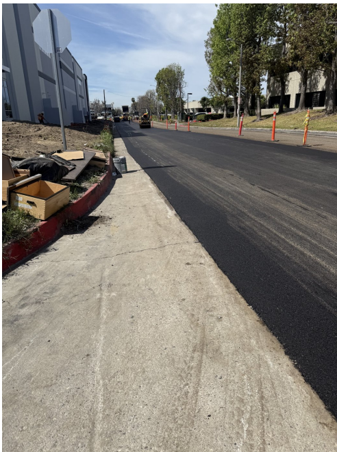
Finished reinforced mat placed in the single-day operation.
