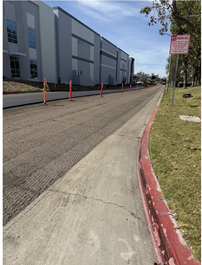
The prepped Lincoln Way alignment ready for the reinforced placement.
