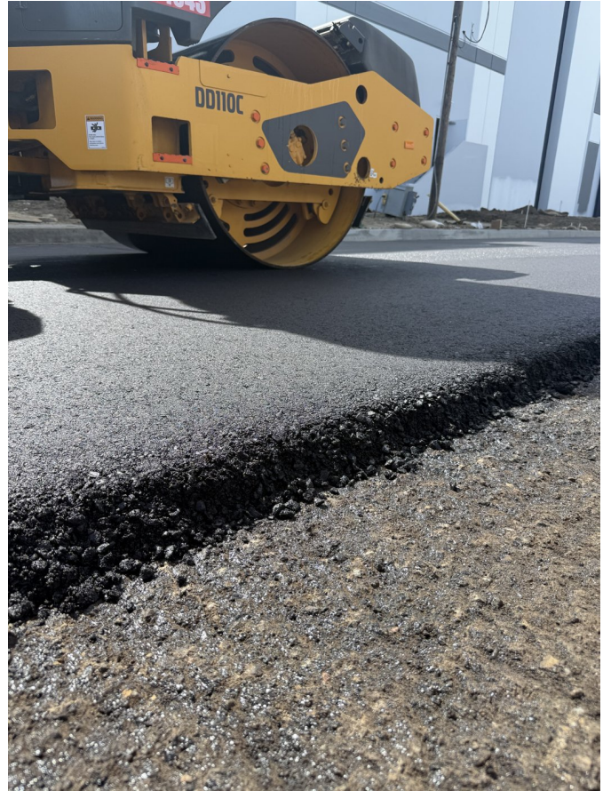
Roller working the fiber-reinforced mat — fresh lift against the milled grade.
