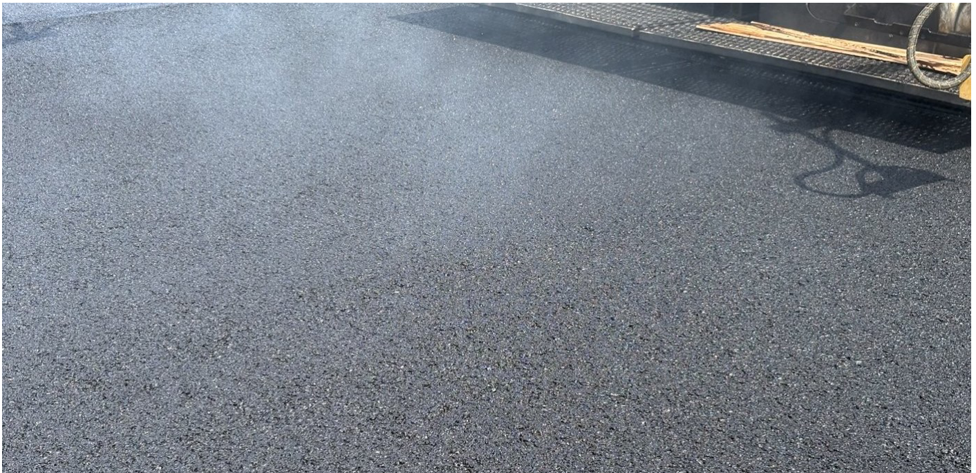
Fresh ACE XP-reinforced mat behind the paver — Market Street, Spokane
