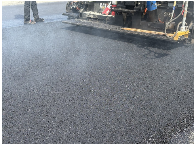
Uniform, well-compacted reinforced mat across the fresh placement.
