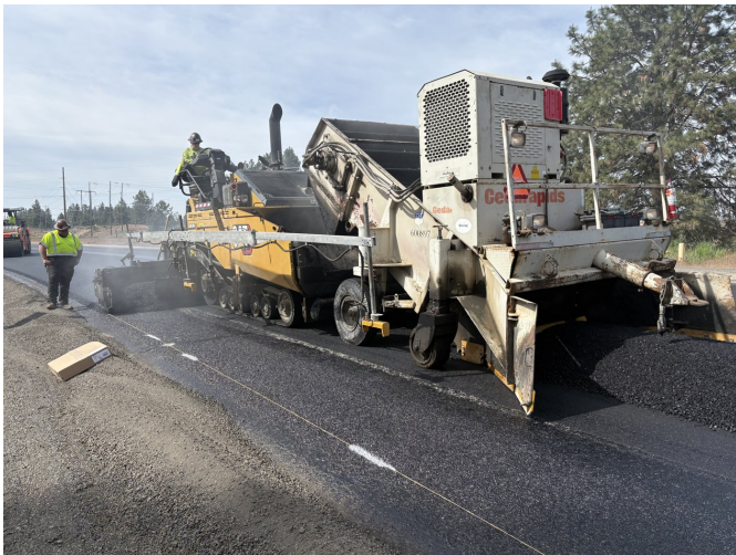
The full paving train at work on the Market Street corridor.
