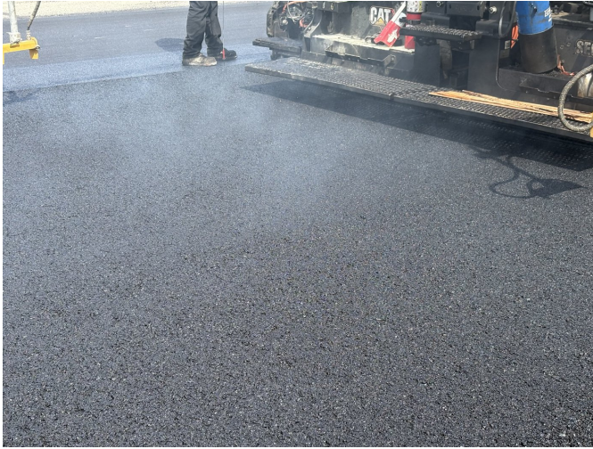
Steaming ACE XP-reinforced mat placed behind the paver.
