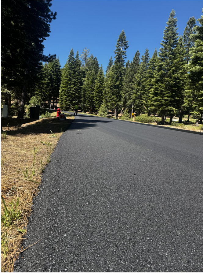
The completed section — built for Sierra winters at 6,000+ feet.
