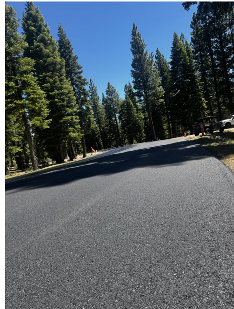
New reinforced pavement winding through the pines at Martis Camp.
