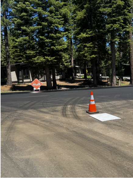
Prepared roadway ahead of the reinforced overlay placement.
