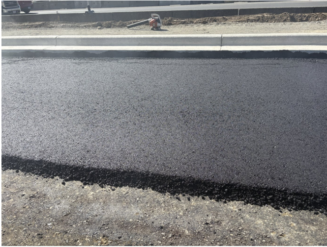
Fresh mat against the new curb line — uniform, tightly bound surface.
