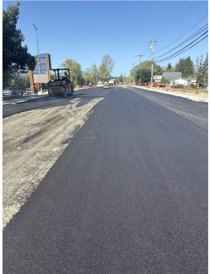
The reinforced corridor taking shape through Port Alberni.
