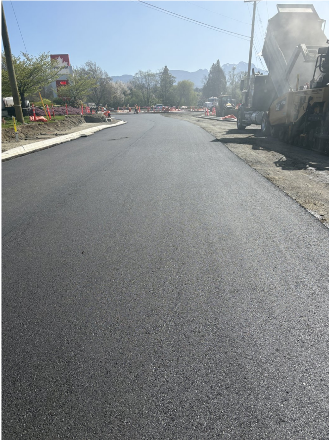
Reinforced pavement placed through the corridor — haul truck feeding beyond.
