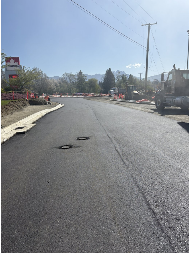
Fresh reinforced mat on the Beaver Creek Road approach.
