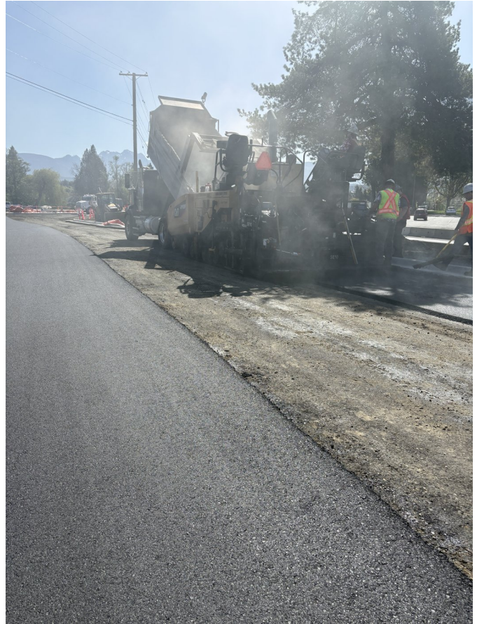
Amrize's paver placing the fiber-reinforced mix.
