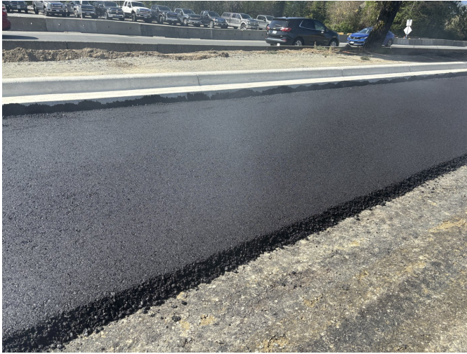
Completed section of the reinforced placement along the new curb.
