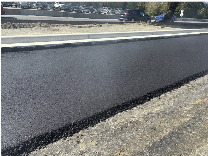
Mat texture detail along the curb transition.
