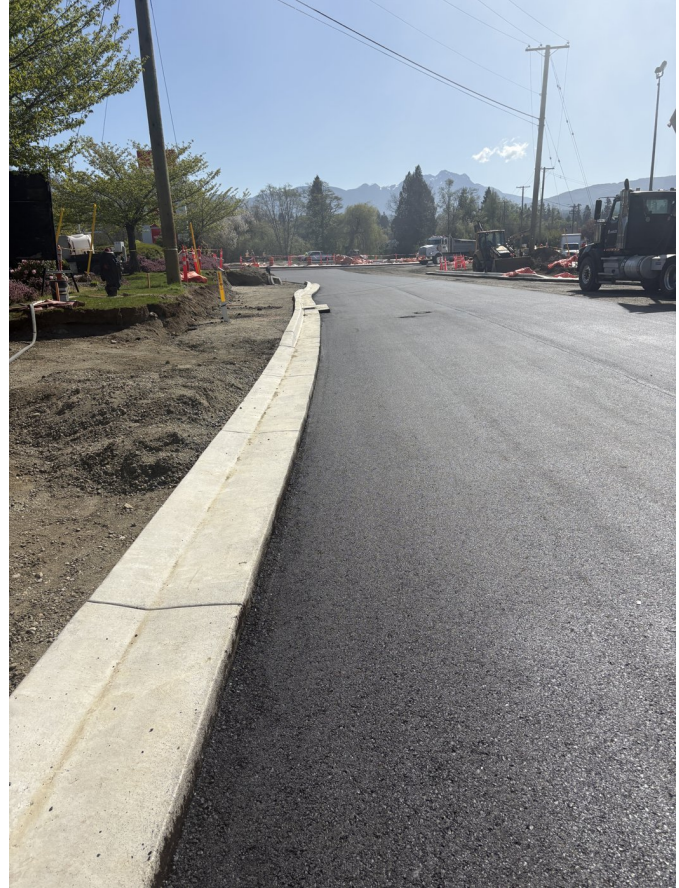
The new ACE XP-reinforced lane against fresh curb and gutter.
