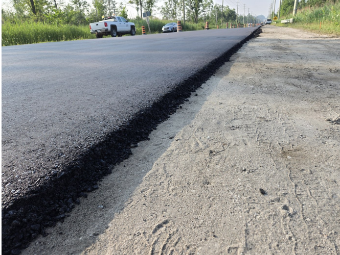
Fresh ACE XP-reinforced mat placed along the CR 27 alignment.
