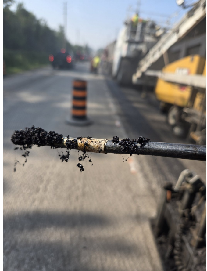
Fiber-reinforced mix on the lute — paving train working behind.
