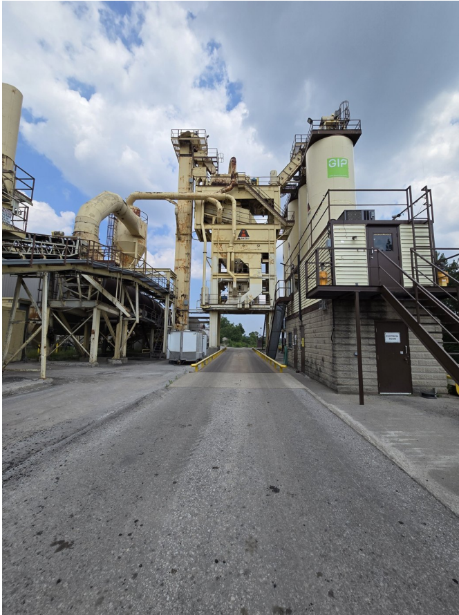
GIP Paving's Barrie plant — production source for the reinforced mix.
