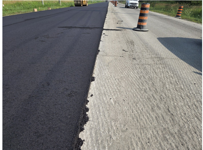
The new reinforced lane under traffic control on County Road 27.
