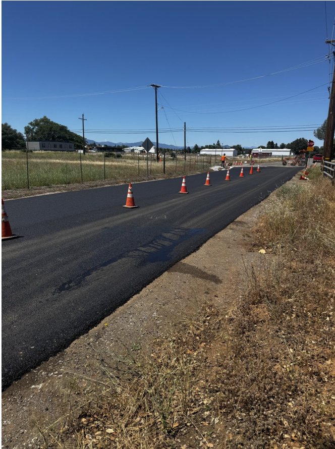
The completed lane under traffic control — single-day placement.
