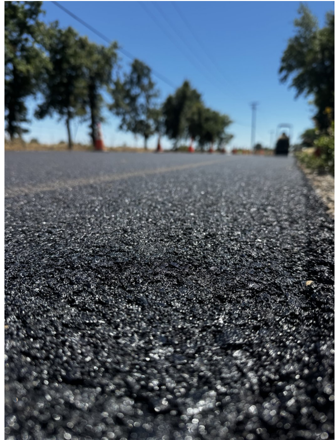
The reinforced overlay looking down the Venture Parkway alignment.
