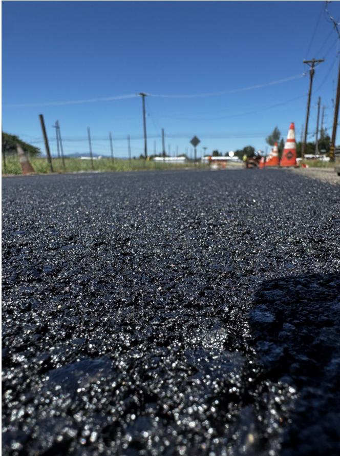
New mat placed at the section approach — crew finishing beyond.
