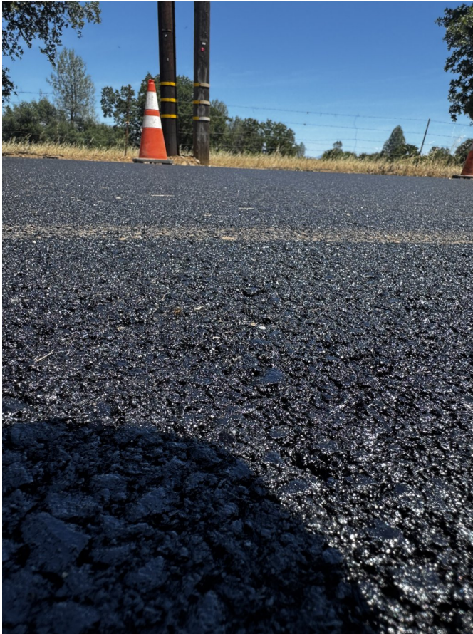
Fresh ACE XP-reinforced mat — tight, uniform texture behind the paver.
